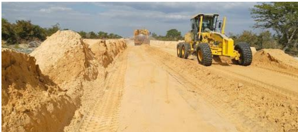
Figure 8 : Construction of the Zambia- Angola International Trade route
